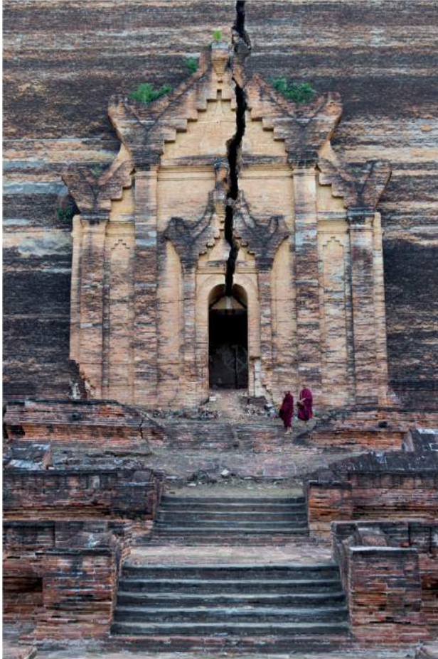
The team's route passed by religious sites such as the Mingun Pagoda, near Mandalay, in central Myanmar. Construction began in 1791. The facade was later split by an earthquake.
